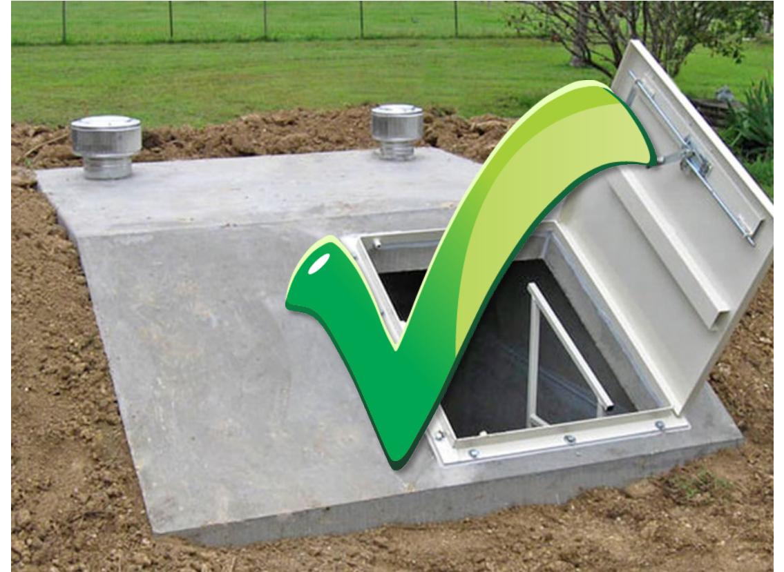
Safe room in tornado country Mitigation
