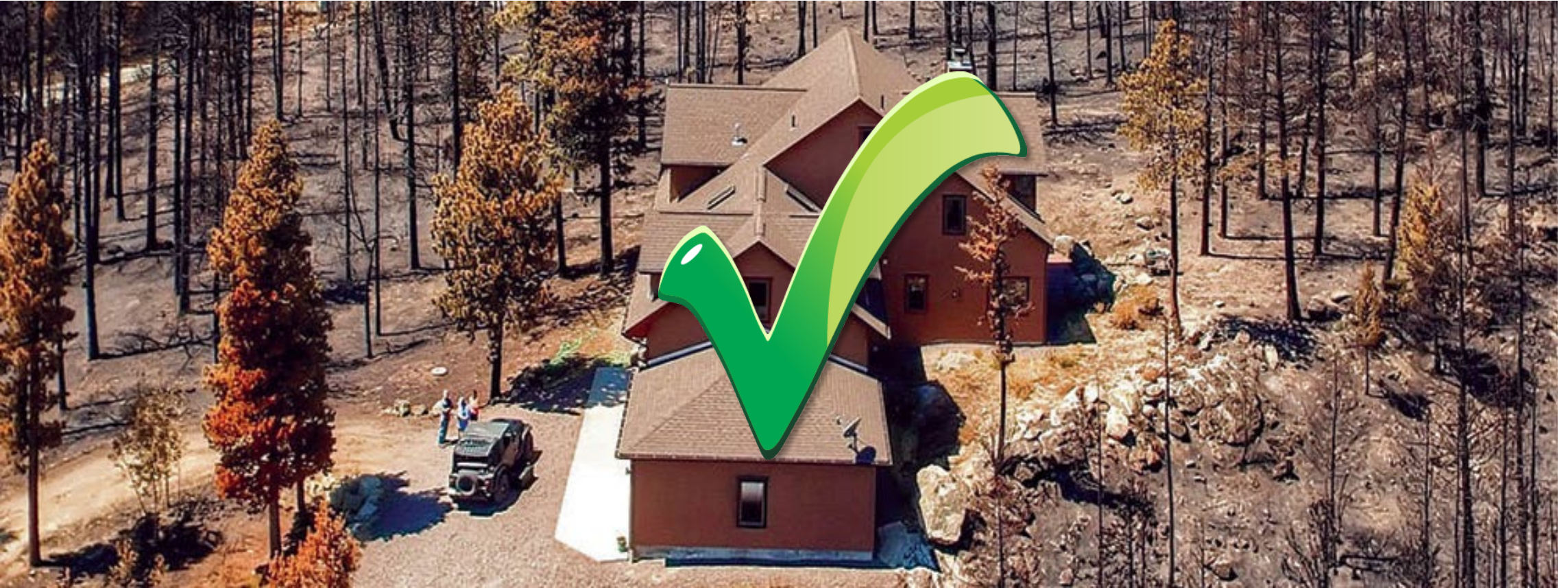
Home hardening and creation of defensible space, Boulder County
