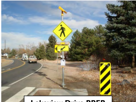
Lakeview Drive RRFB
