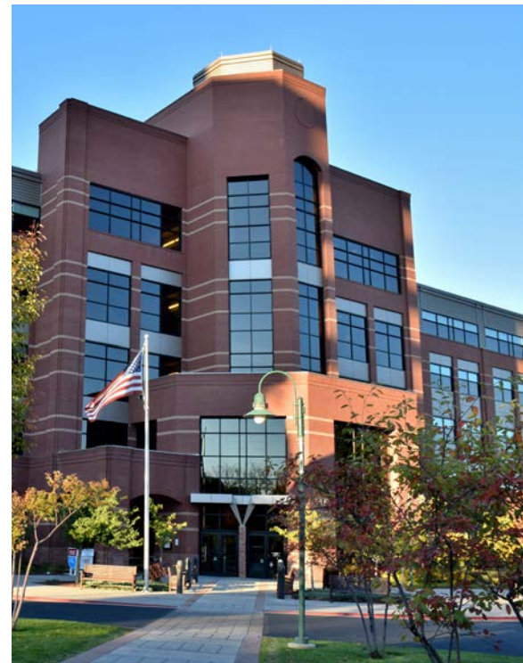
Larimer County Building. Photo: Alisha Jeffers
