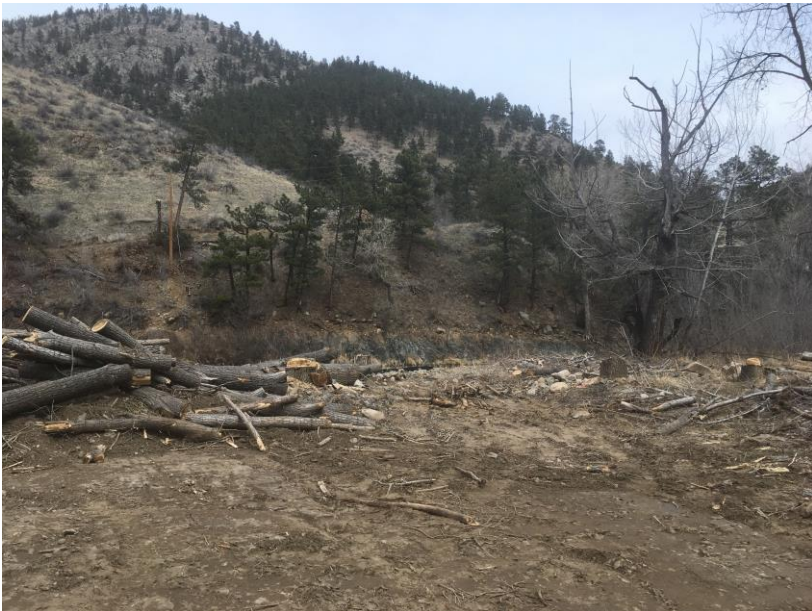
The Narrows – Hazard Tree Removal
