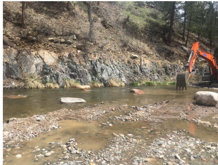
Boulder placement, April 2019
