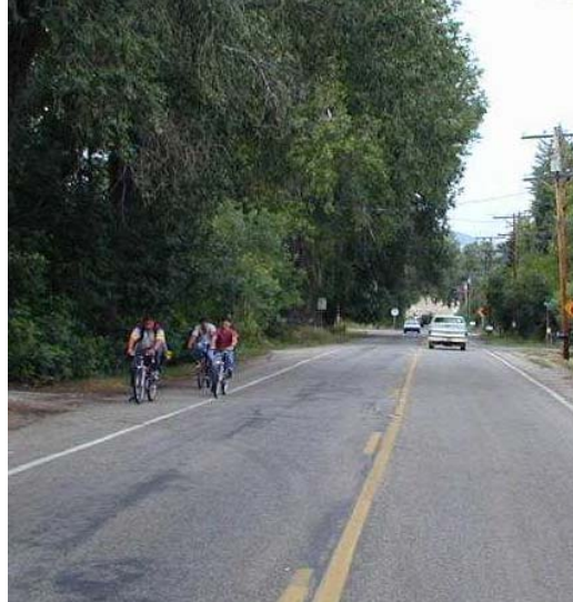
Narrow Shoulders for Bicycling
