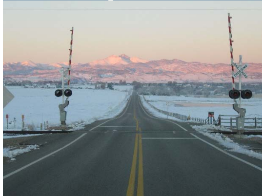
Railroad Crossing with Gates & Flashers
