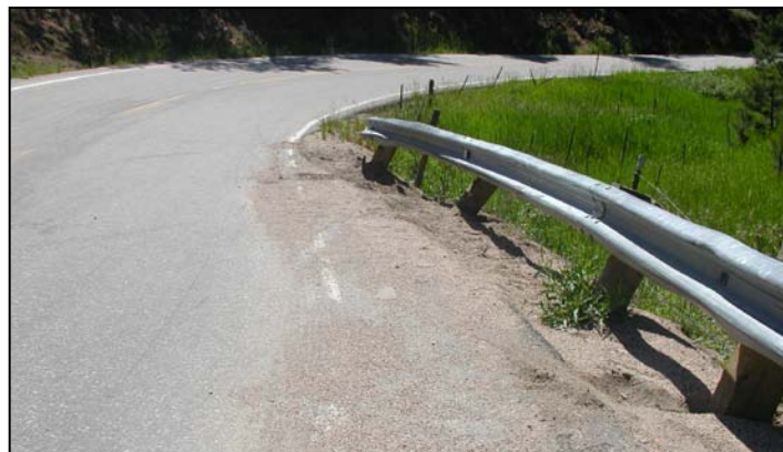
Damaged Guardrail on CR 27. A realignment project will further enhance safety.
