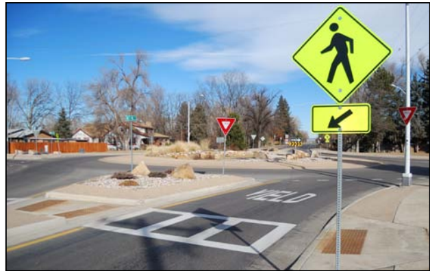
Roundabout at CR 19 (Taft) / CR 48 (Vine)
