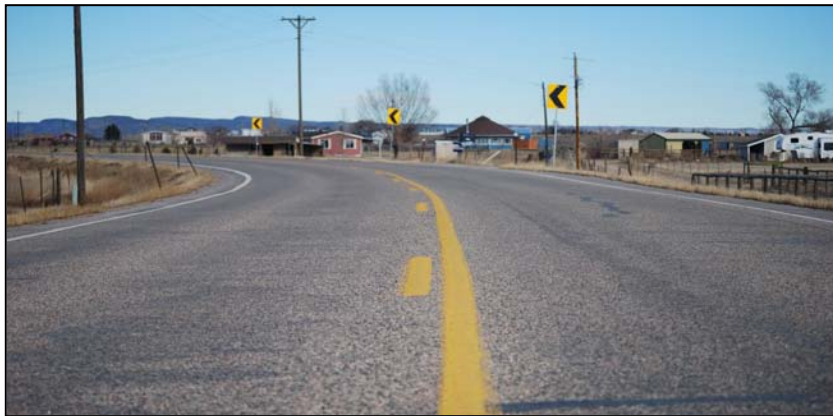
Chevron Signs on CR 19 S-Curves north of CR 60E
