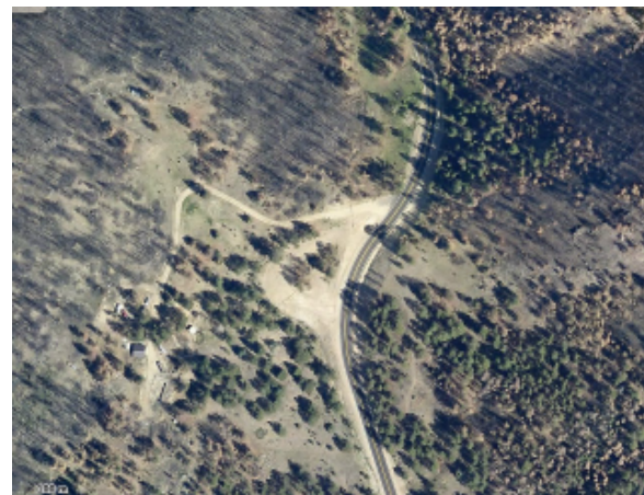
CR 27 after realignment
