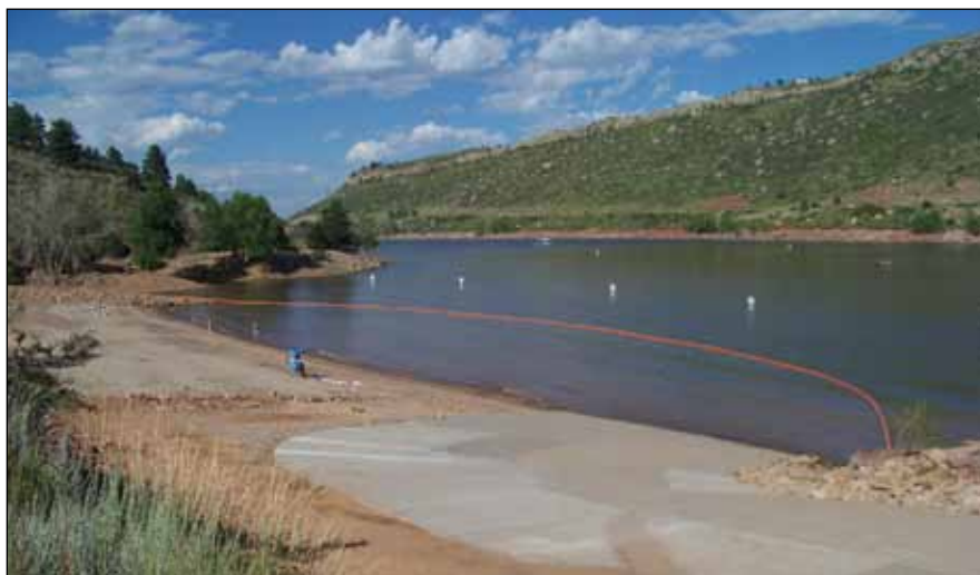
Horsetooth Reservoir County Park swim beach construction at high water. Photo: Gary Buffington
