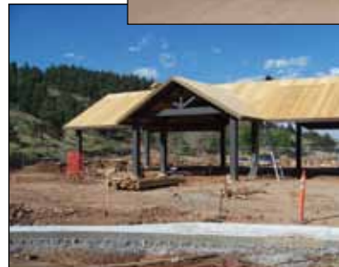
Group pavilion under construction at Horsetooth Reservoir. Photo: Gary Buffington
