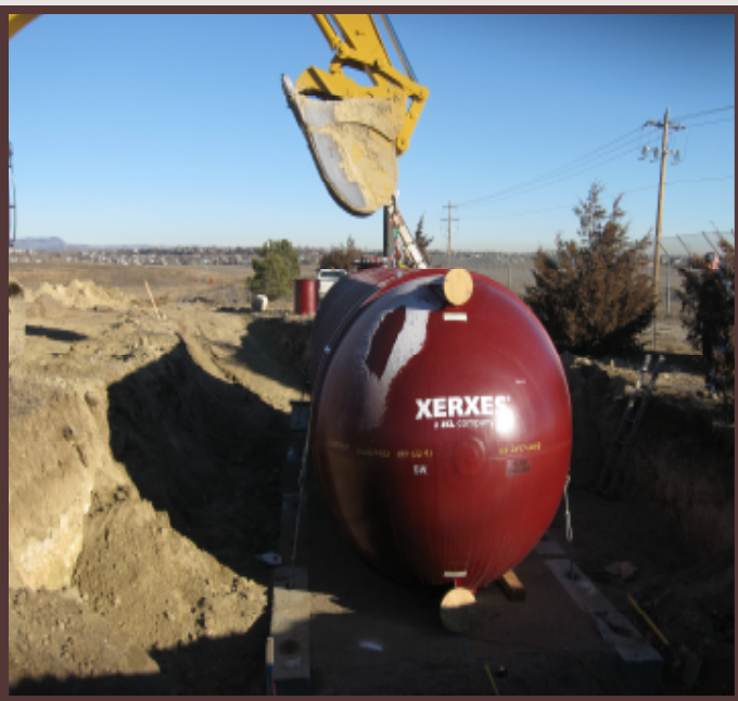
A new 12,000 gallon underground water tank was installed last year.
