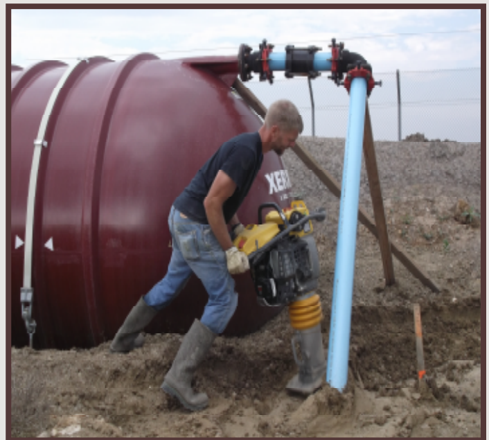
Construction of new water filling station for dust mitigation took place in 2015.
