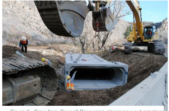
Figure 5: Crew from Connell Resources places new culvert along Rist Canyon Road. Photo by Pamela Dickman/Herald Staff Writer
