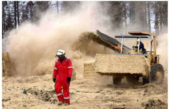
Figure 16: Post-fire mulching for runoff and erosion mitigation
