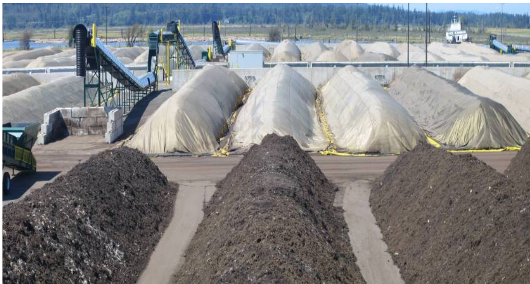
Figure 10-1. Example of an Aerobic Composting Facility – Forced Aerated Static Pile
