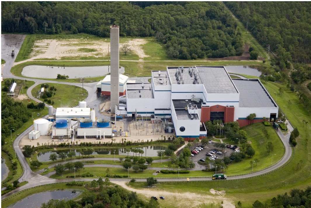
Figure 8-1. Aerial View of Lee County WTE Facility in Fort Myers, Florida
