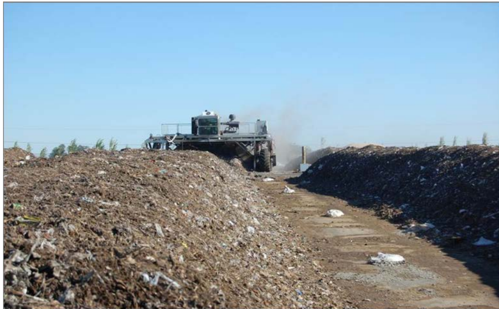
Figure 6-1. Example of a Windrow Aerobic Composting Facility
