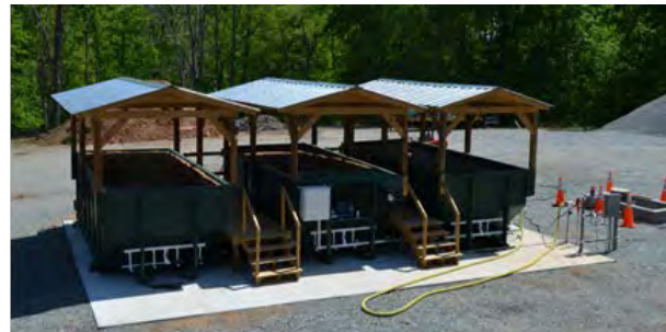
Aerobic Composting Including Food Waste
