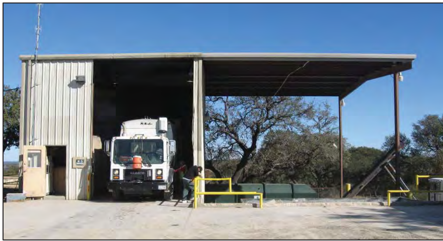
Figure 3-4: Example of Compactor Transfer Station
