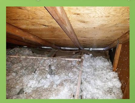
Hot spots at every soffit vent are very common, especially in windy areas.
