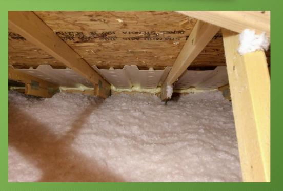
Spray-foam at bottom of soffit-vents secures baffle and better isolates ventilation from insulation.
