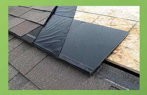
Provides ample, and continuous ventilation to match ridge-vent,
