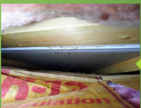
Looking down from the top of the knee-wall, at gaps between drywall and insulation:
