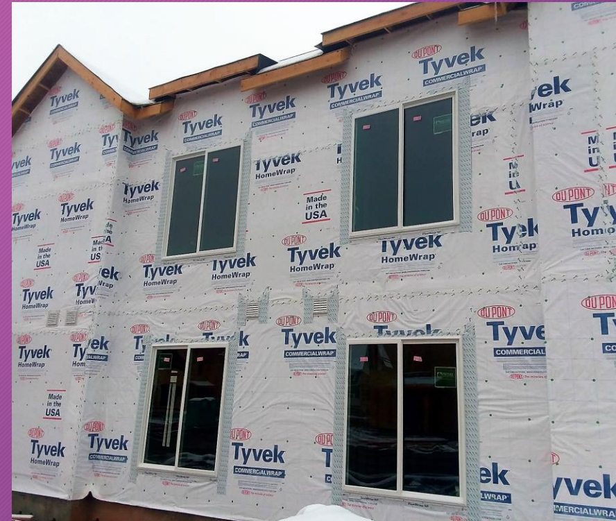
Above: Properly integrated & flashed
