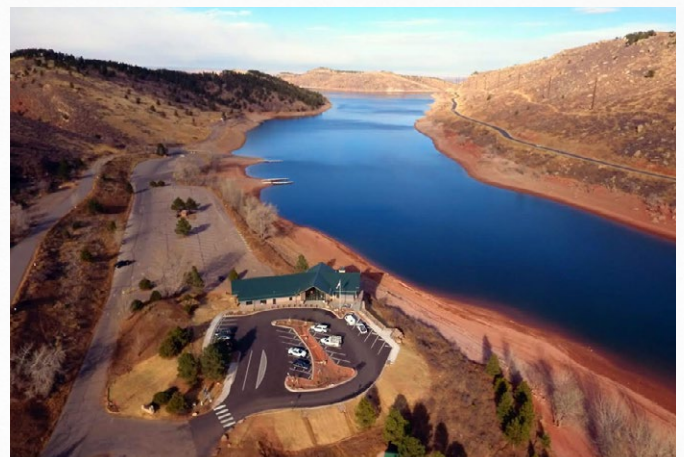
Horsetooth and Carter Lake reservoirs road and parking improvements
