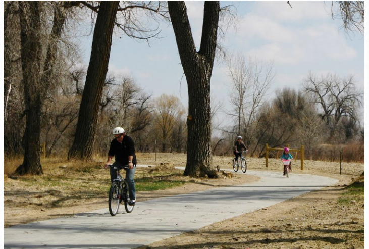
Poudre River Regional Trail Construction
