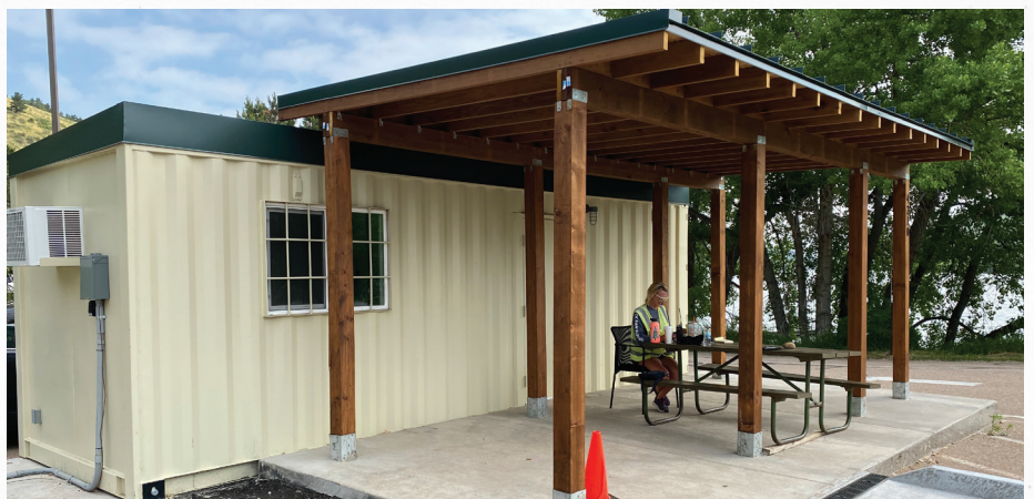
A newly completed ANS station offers shade and a protected place for staff to shelter out of the elements, if needed.
