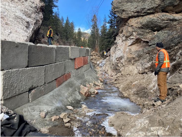
Photo 6 - Completed concrete block wall
