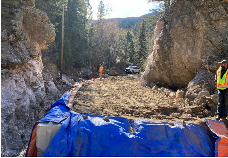
Photo 5 Pinch point looking downstream
