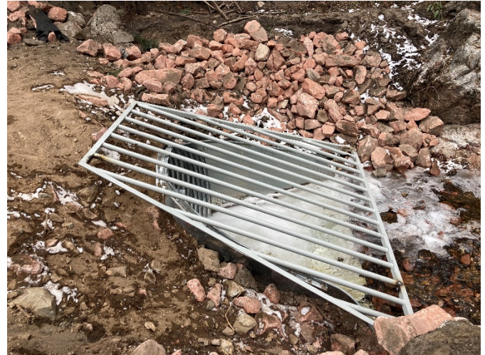
Photo 1 - Copper Hill Road trash rack
