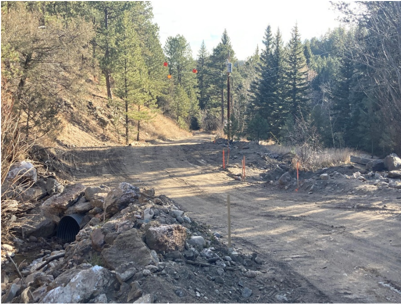
Photo 4 - 635 Streamside Dr overtopping structure
