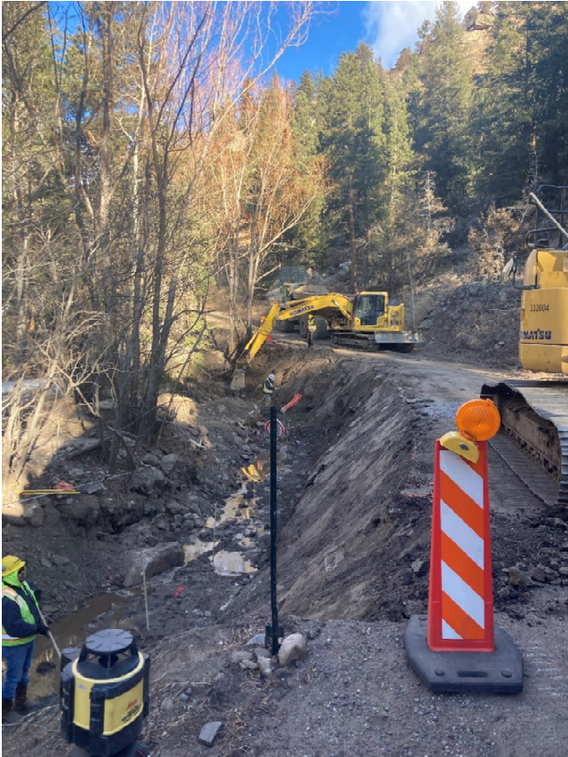
Photo 3 - Streamside Dr revetment
