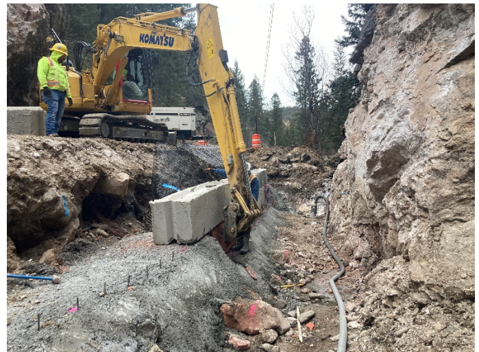
Photo 2 - Constructing the concrete block wall at the pinch point
