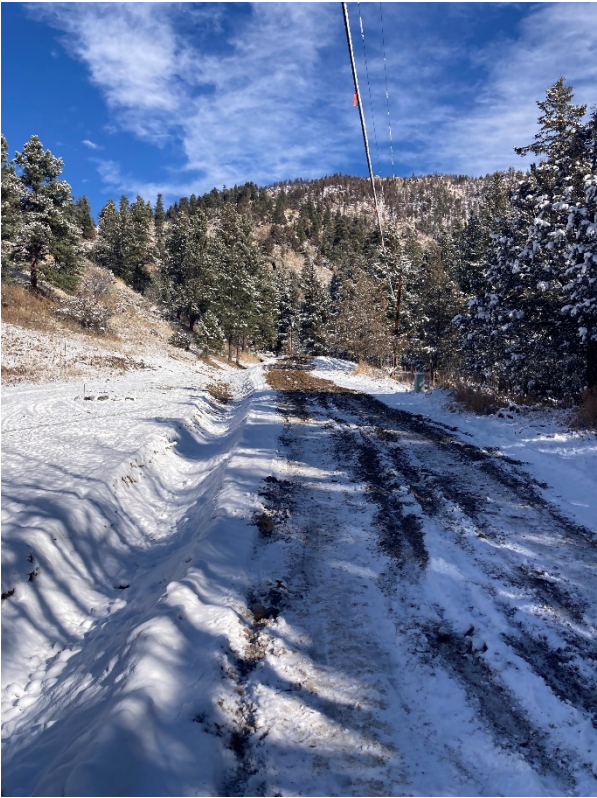
Photo 4 - Roadside swale on upper Black Creek Drive
