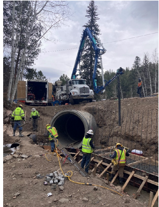
Photo 1- Upper Streamside upstream footers
