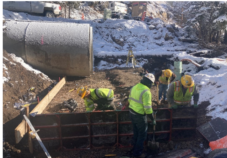
Photo 2- Upper Streamside downstream footers
