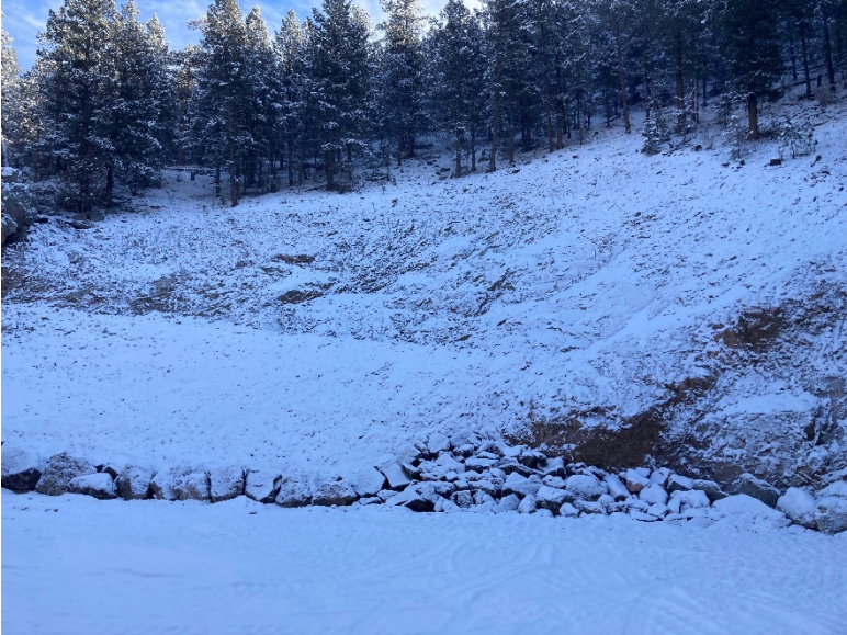
Photo 6 - Borrow site after final grading
