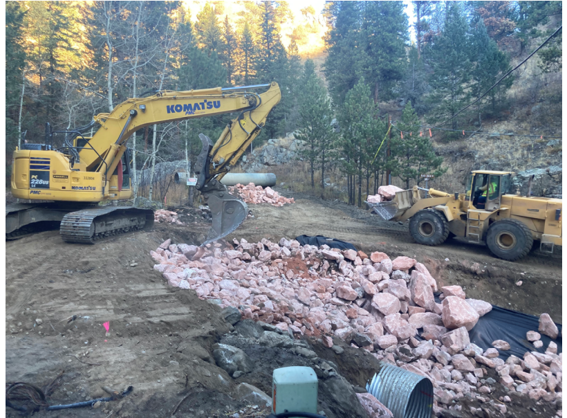
Figure 1- New 60" cmp and riprap at Copper Hill Rd
