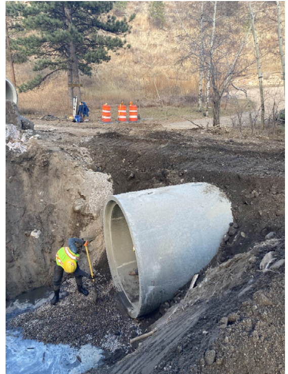
Figure 1- New 84" RCP at lower Streamside Crossing
