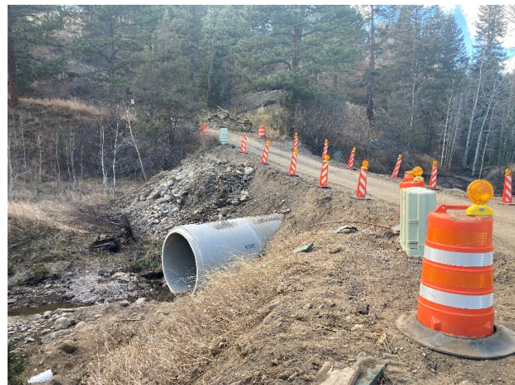
Figure 2- Upper Streamside 84" RCP
