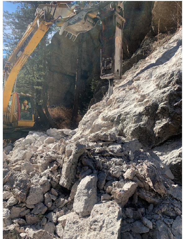
Photo 1- Widening the pinch point on Black Creek Drive
