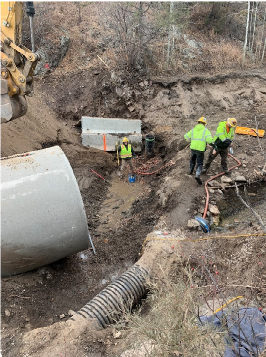
Photo 5 - Preparing to form wingwalls/headwalls on upper Streamside culvert
