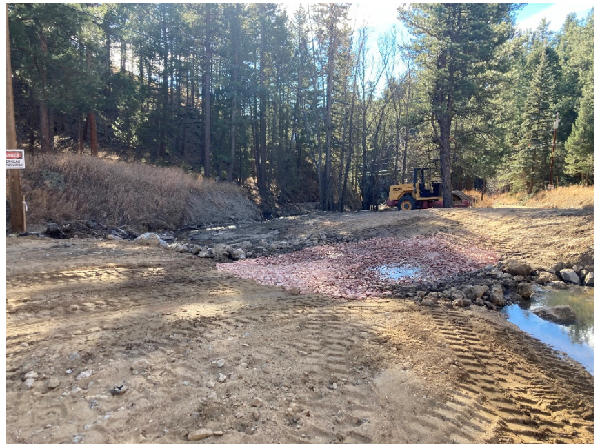
Photo 6 - Black Creek Dr low water crossing
