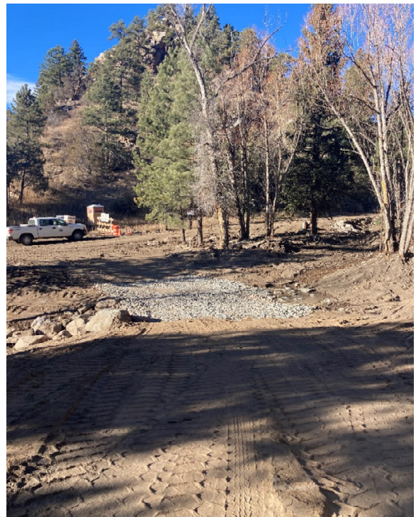
Photo 2- Corner Court low water crossing
