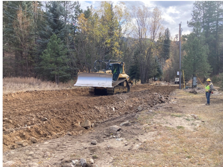
Figure 2- Placing material from borrow site in Black Creek Drive
