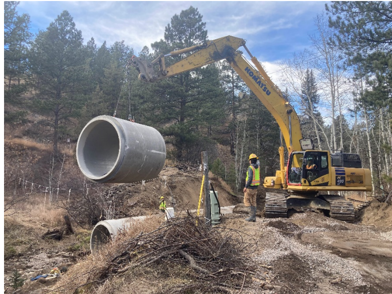
Figure 1- New 84" RCP at upper Streamside Crossing
