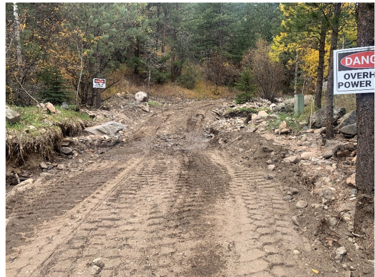
Figure 2- Temporary low crossing to keep water in original alignment
