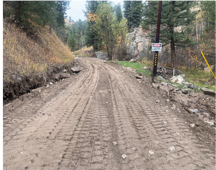
Figure 1- Primitive Road to provide access to entire project length
