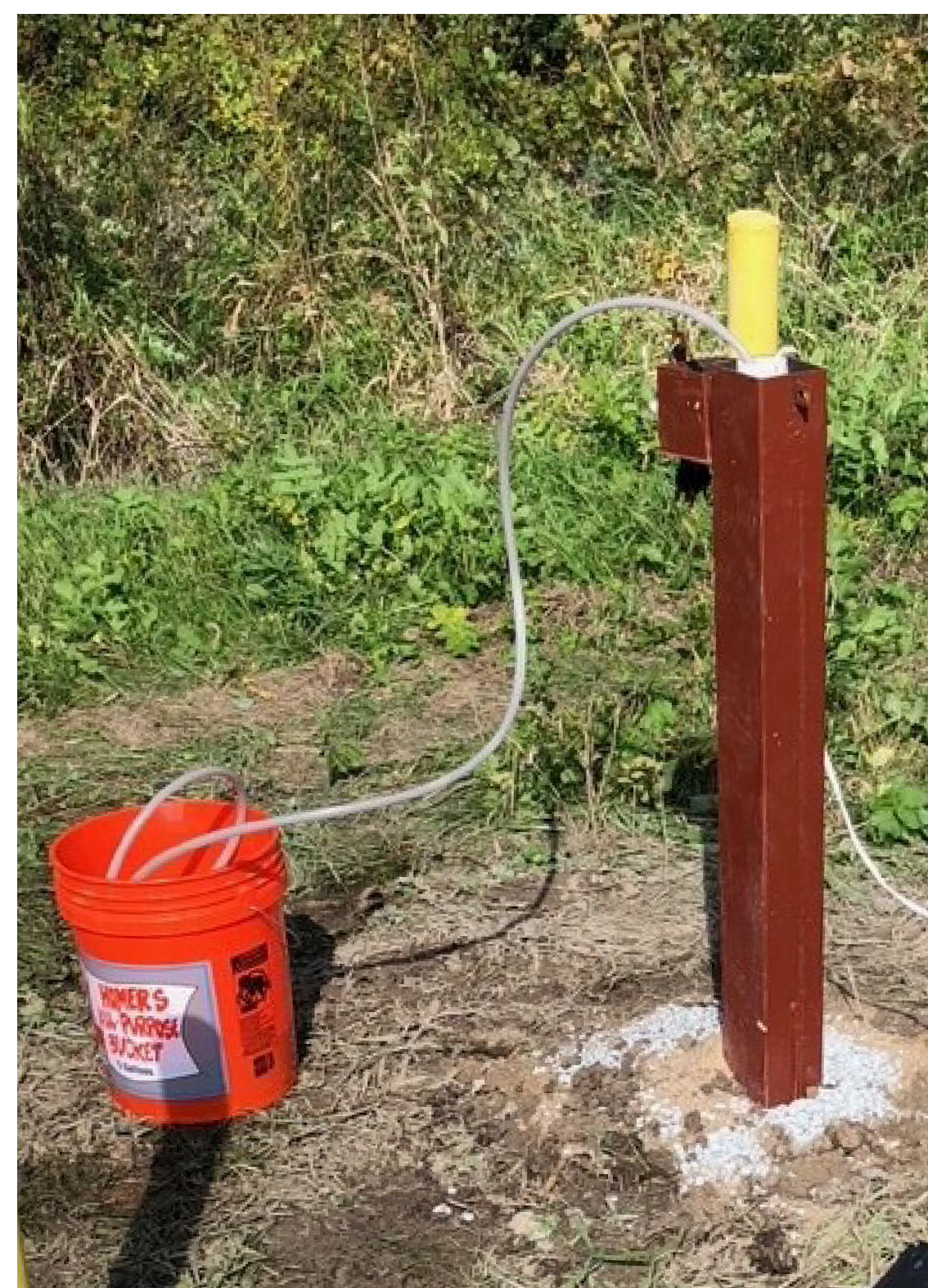
Groundwater monitoring well.
