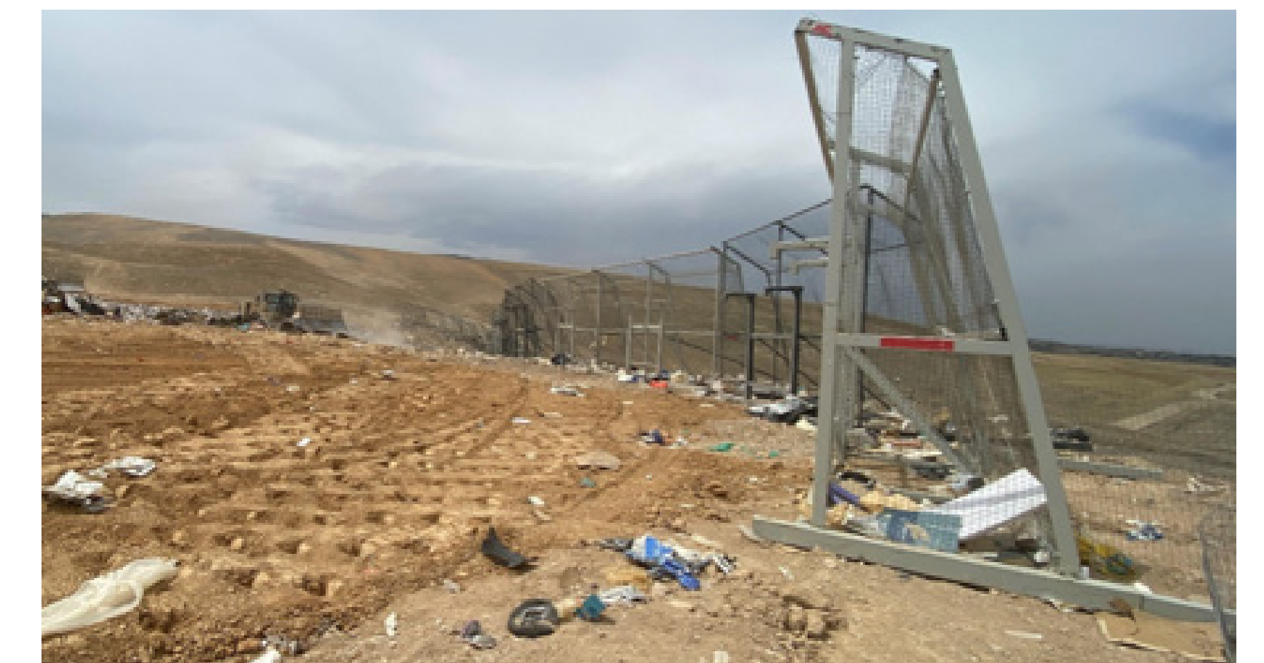
Portable panel fencing near the working face.
