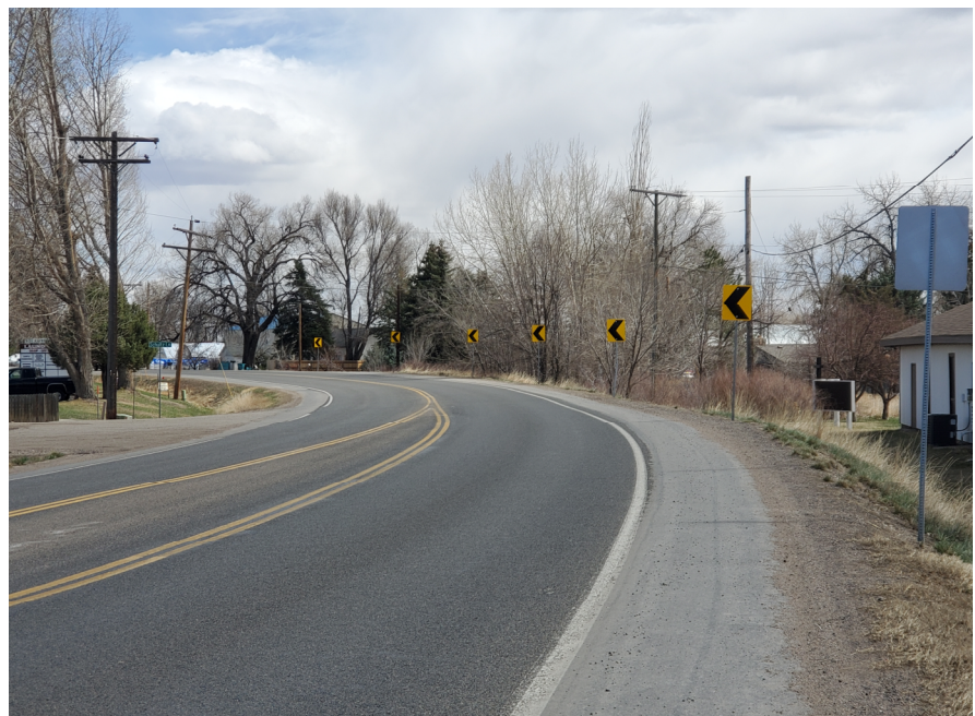
Chevron signs installed on CR 54G west of Indigo Hills Ln
