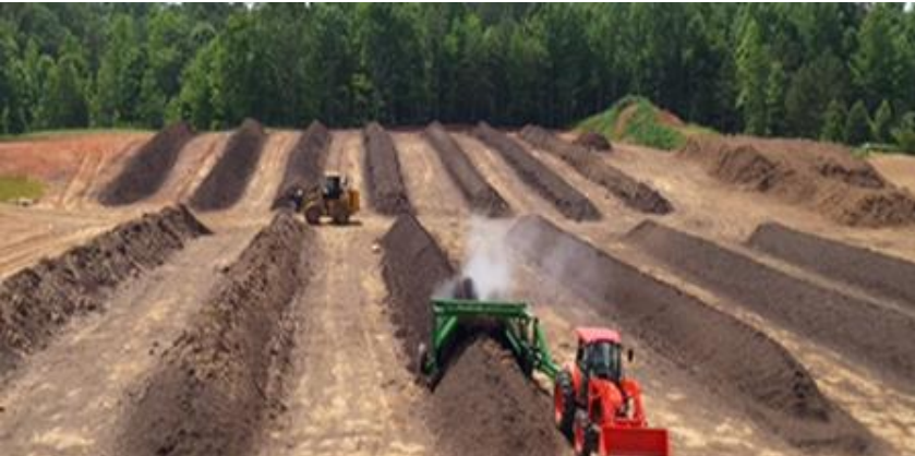
Yard Waste Organics Processing Facility
