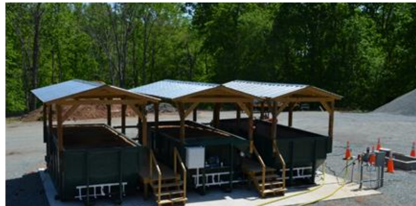
Aerobic Composting Including Food Waste
