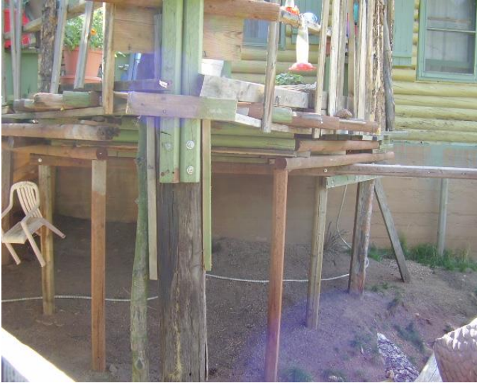
Unsafe deck beams, posts, footings, and rails.
