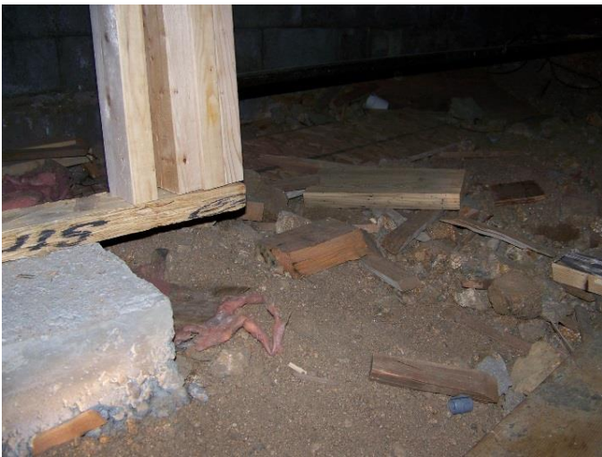
Missing point loads in the crawl space
