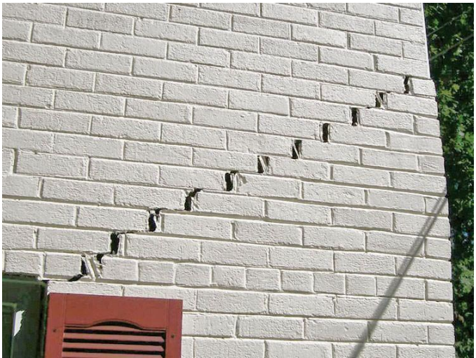
Stair-step cracking
