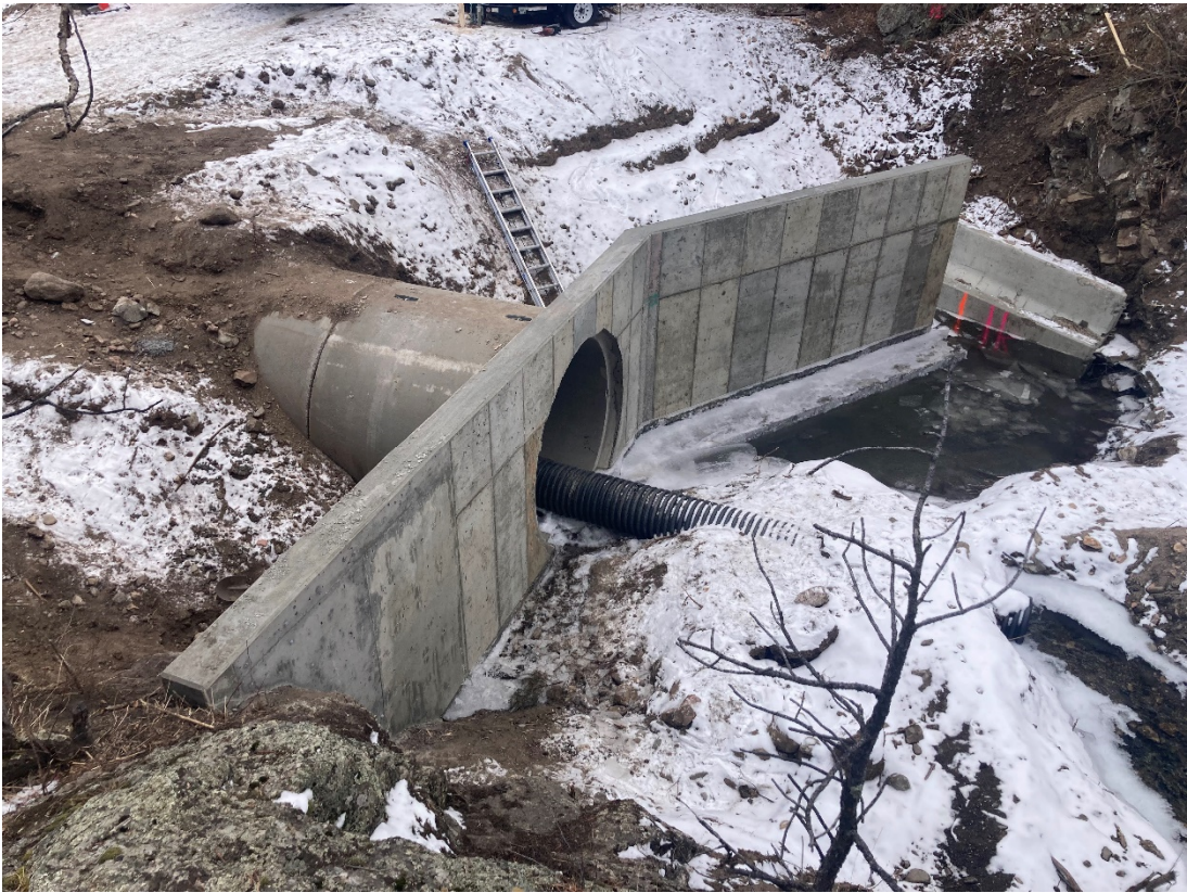
Photo 3- Upstream end of Upper Streamside Drive
