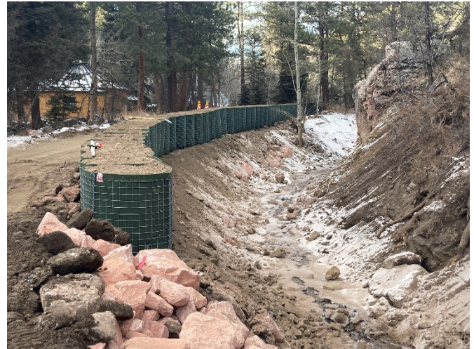
Photo 1- Flood barrier bags along Streamside Drive
