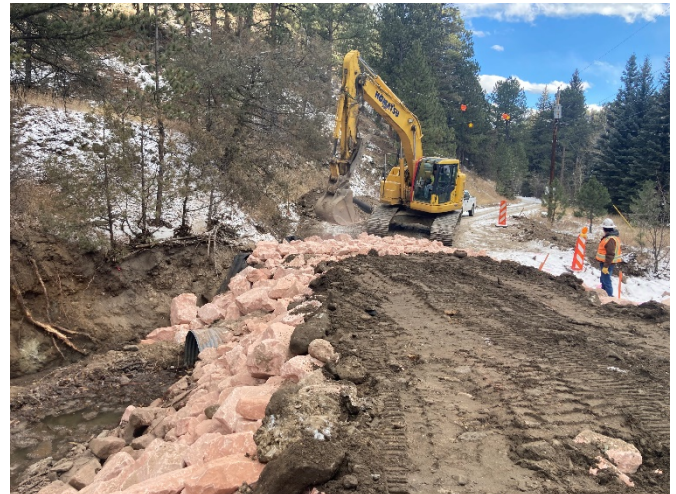
Photo 2- Constructing Streamside Drive overtopping structure
