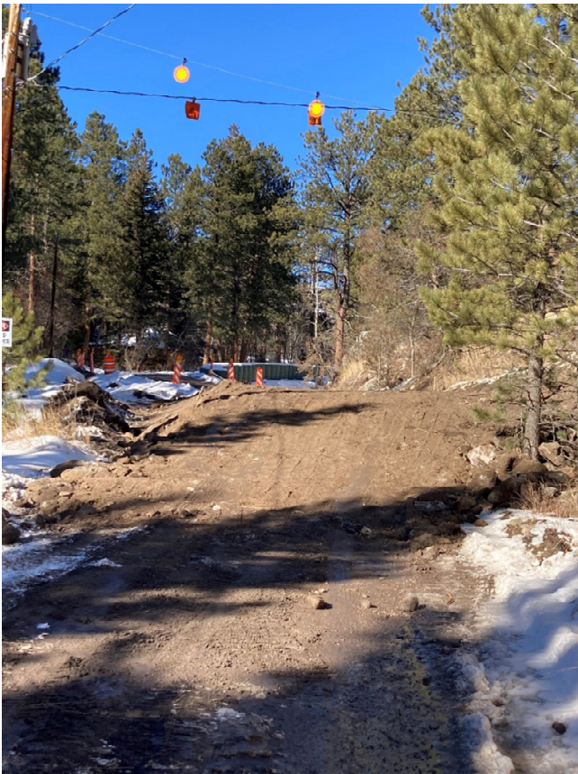
Photo 3- Overtopping structure upstream of the confluence
