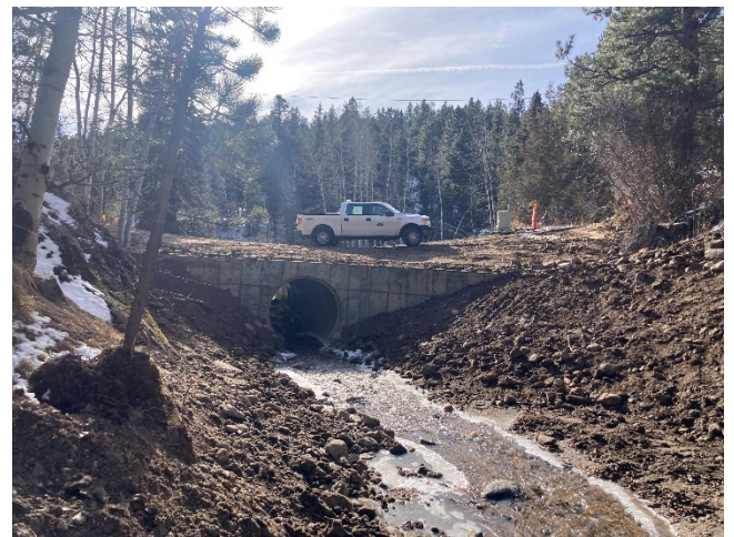
Photo 2- Completed upper Streamside crossing
