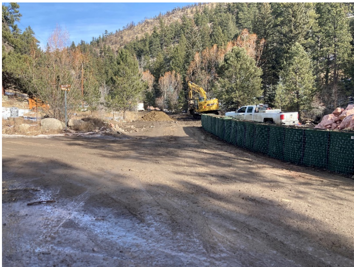
Photo 5 -Flood barrier bags leading into Black Creek Dr
