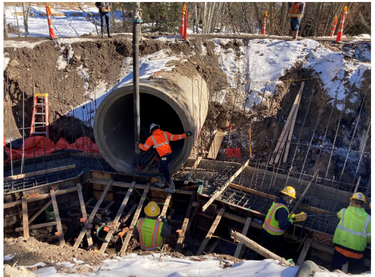
Photo 4- Pouring lower Streamside footers
