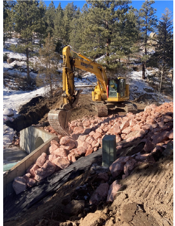
Figure 1 -Installing 24" riprap on upper Streamside
