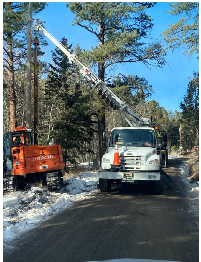
Photo 6- Estes Power setting new poles
