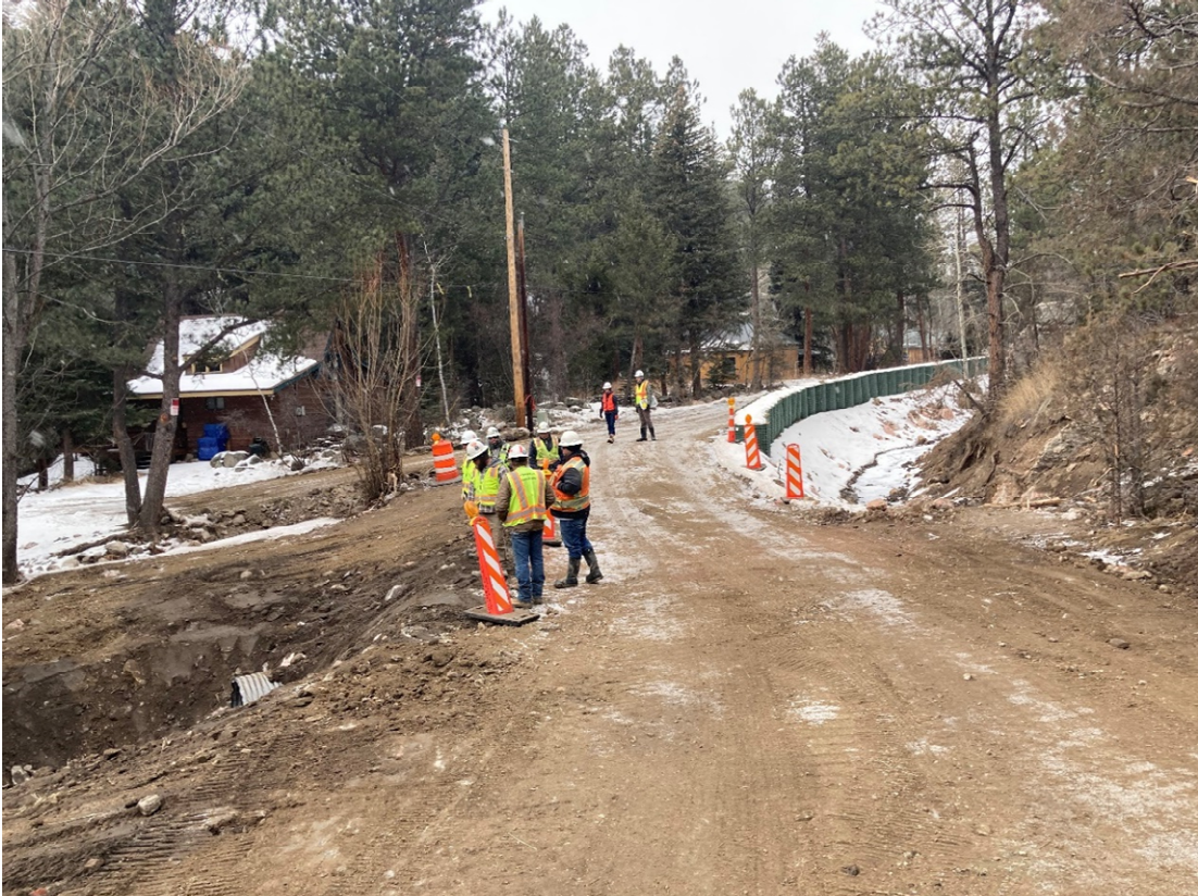
Photo 3-Streamside Dr overtopping structure upstream of the confluence
