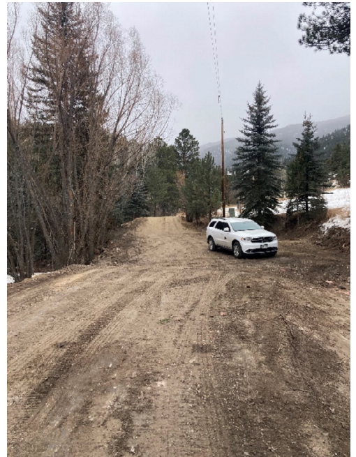
Photo 2 - Lower Streamside overtopping structure
