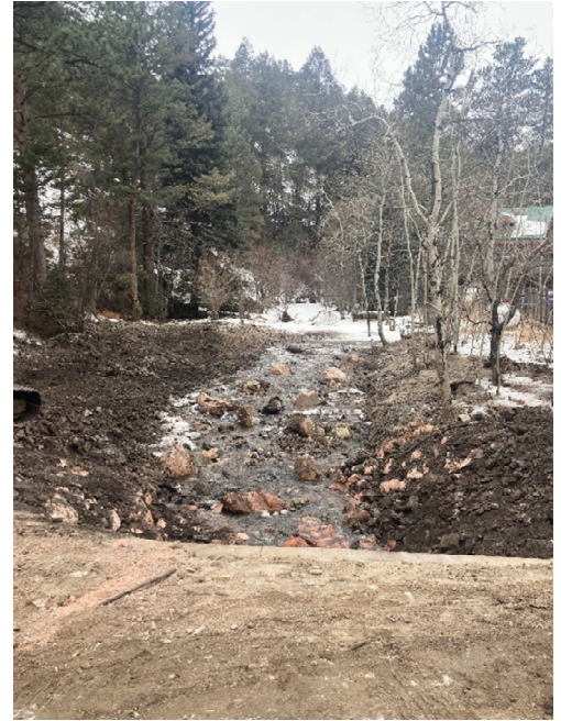
Photo 1 - Riffle above lower Streamside Culvert
