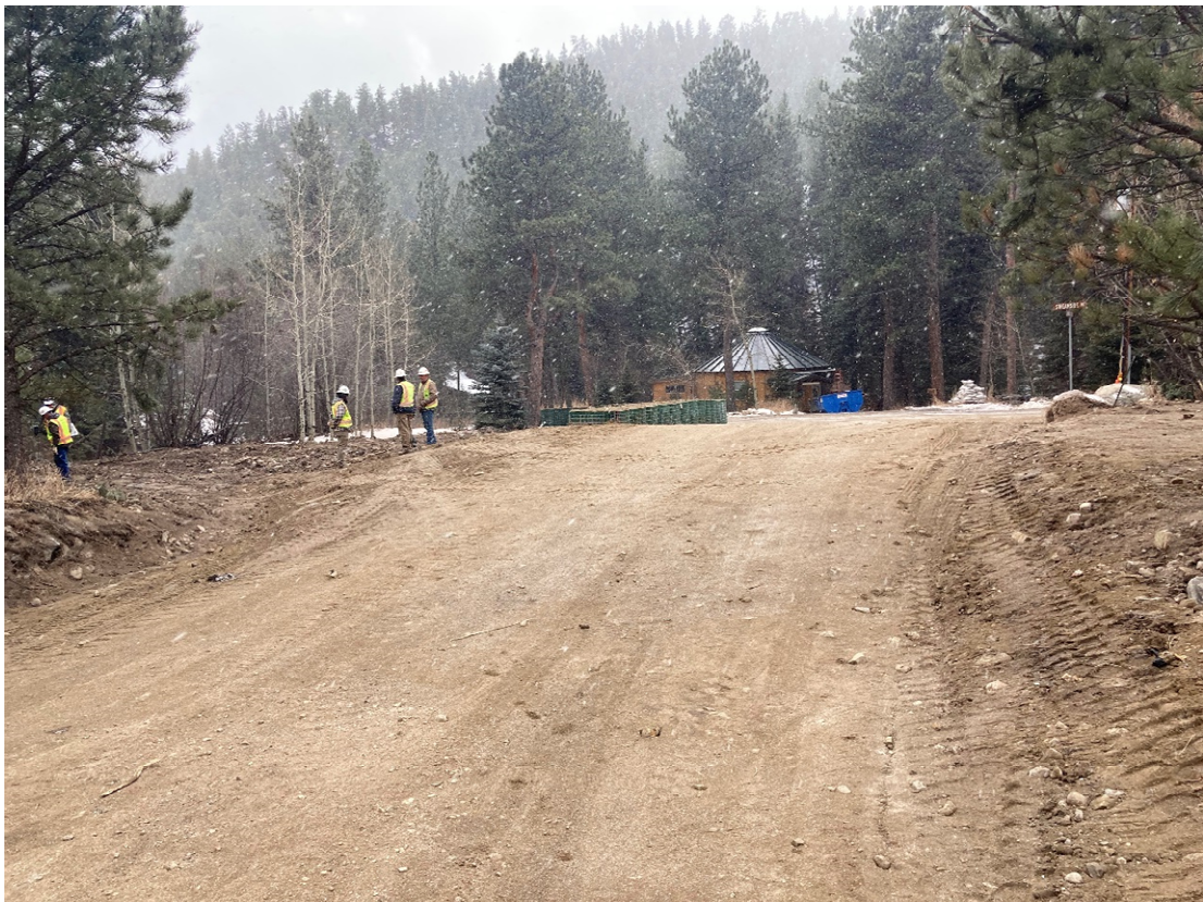
Photo 4- Lower Black Creek Drive water bar
