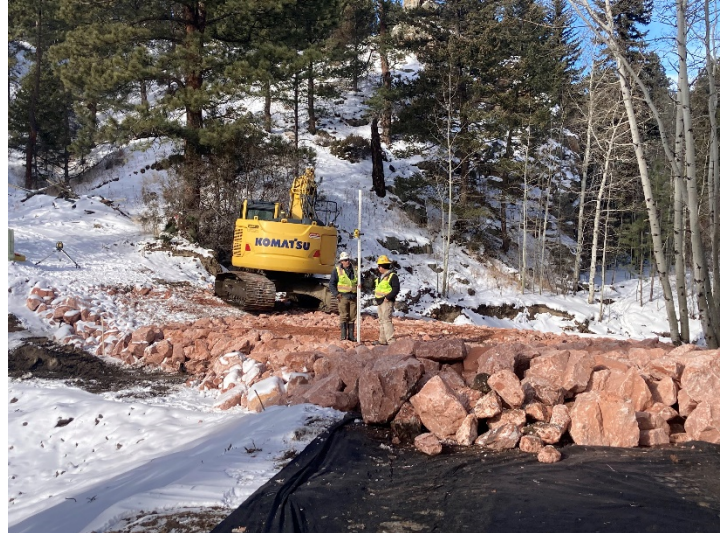
Photo 1- Checking grades on Upper Streamside Drive Overtopping Structure
