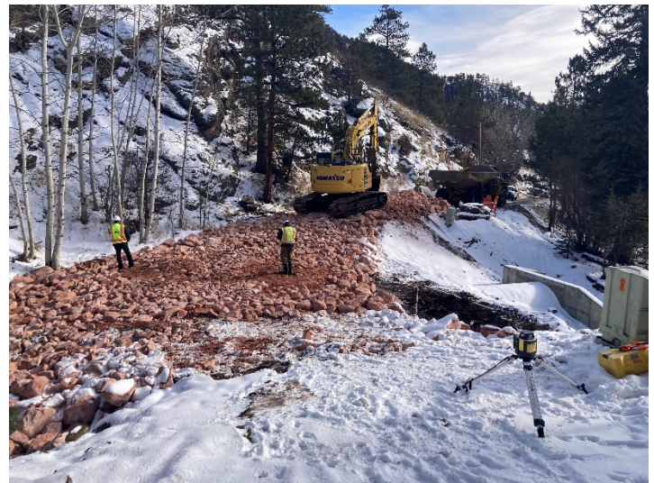
Photo 2- Constructing Upper Streamside Drive overtopping structure
