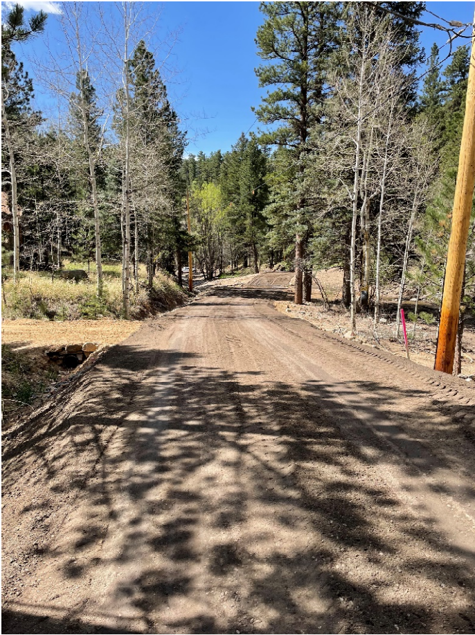
Installed Recycled Asphalt on Black Creek Drive
