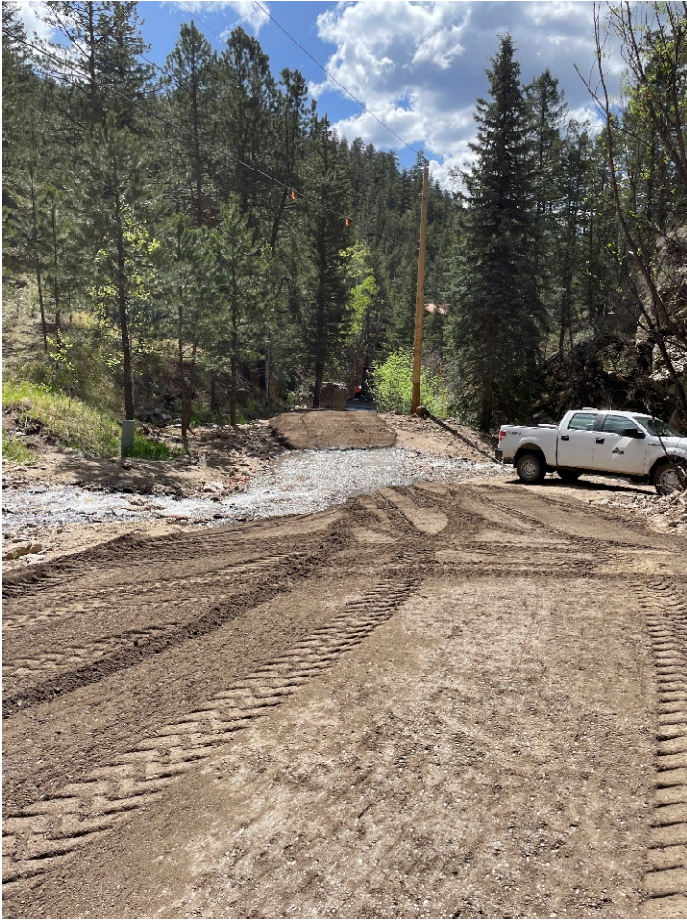
Installing Recycled Asphalt on Black Creek Drive
