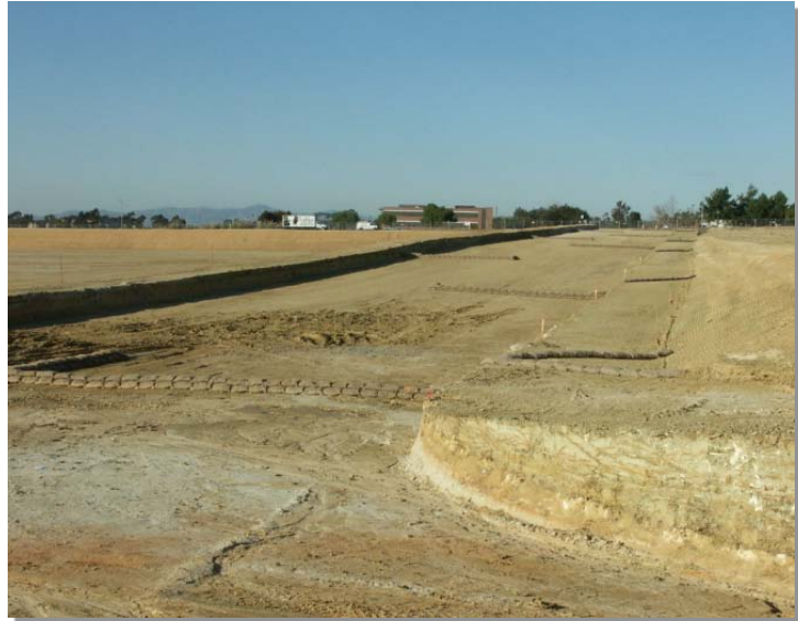
Photograph RCS-1. Rough cut street controls.
