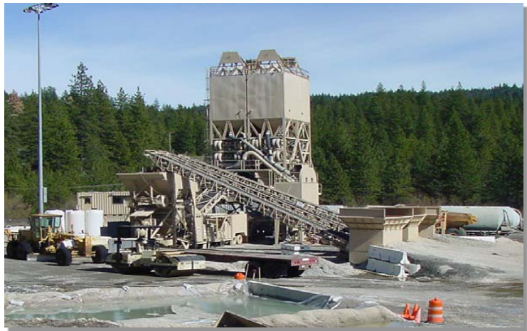
Photograph TBP-1. Effective stormwater management at temporary batch plants requires implementation of multiple BMPs. Photo courtesy of California Stormwater BMP Handbook.
