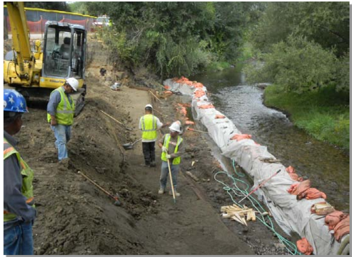
Photograph TDM-1. This coffer dam, installed to allow grading and stabilization of the stream bank, consists of concrete blocks covered by an impermeable liner held in place by sand bags.
