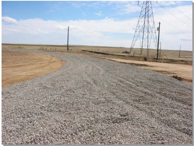
Photograph SCR-1. Stabilized construction roadway.
