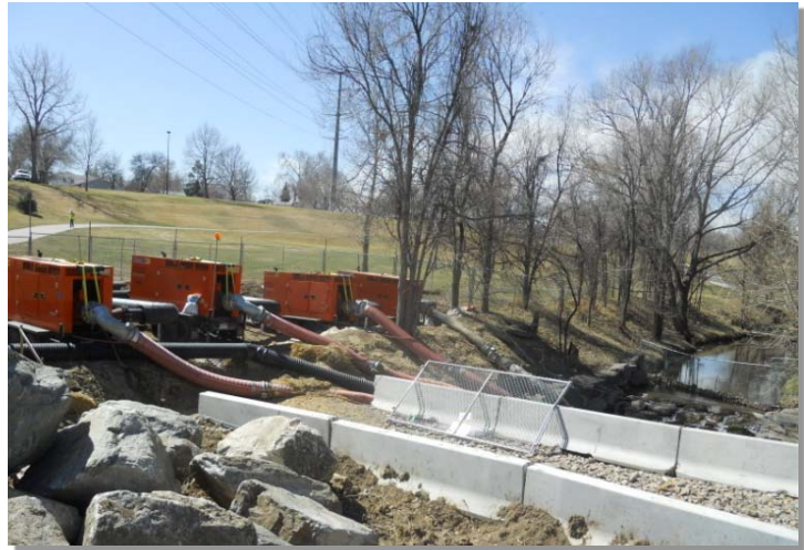
Photograph TDM-2. Despite a relatively significant baseflow, a pumped diversion was selected for this Lakewood Gulch project due to a lack of space crossing Federal Boulevard. Photo courtesy of City and County of Denver.
