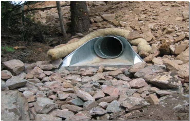
Photograph TOP-1. Riprap outlet protection.
