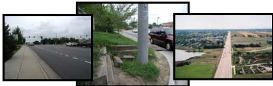
It was noted in the EOS process that the cross-sections for principal arterials used by both cities would equate to a 45 mph design/posted speed. However, as an intra-city corridor, the desire of CDOT and each jurisdiction is to accommodate the existing 55 mph speed limit on US 287 until such time that development and traffic require changes.
