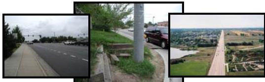
can be developed at intersections as part of signal timing and turn-lane improvements. The widened roadway will have curb and gutter on both sides and will be designed for 55 miles per hour (mph) north of 57<sup>th</sup> Street and 45 mph south of 57<sup>th</sup> Street.
