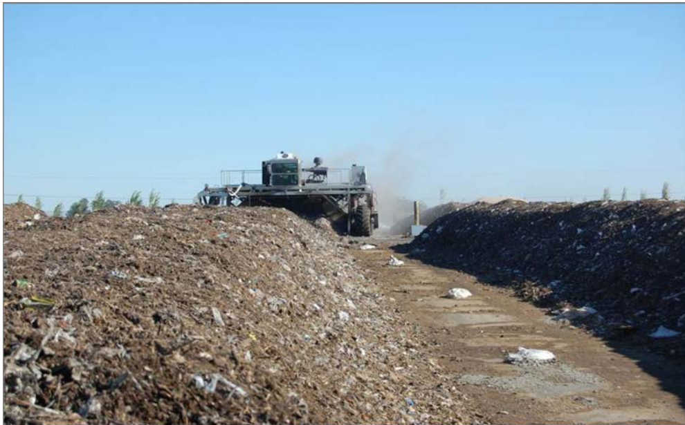
Figure 6-1. Example of a Windrow Aerobic Composting Facility
